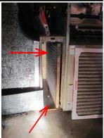
42. Basement utility room Heating System Humidifier: The humidifier is disconnected and non functional.
