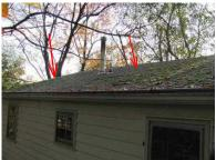
2. Plumbing Vents: Replace all plumbing vent pipe flashing when the roof shingles are replaced.
