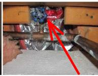
9. Gas Meter: Paint the pipes by the rear gas meter to prevent further corrosion of the pipes.
