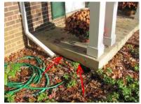
7. Deck: Pressure Treated wood - The rear deck stairs to the back yard have a loose stair tread near the ground level, this is a trip hazard.
