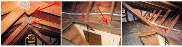
19. Attic Ventilation: Gable vents only. Recommend installing ridge vents and an attic fan to increase attic ventilation.
